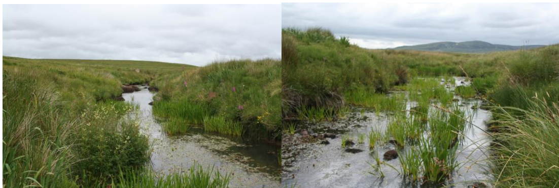
Plate 1-2: Overhead Line Crossing Location of Gowlan River
